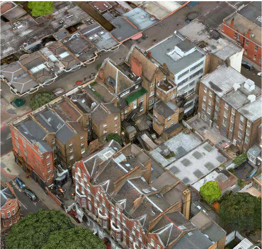
AERIAL: VIEW WEST
