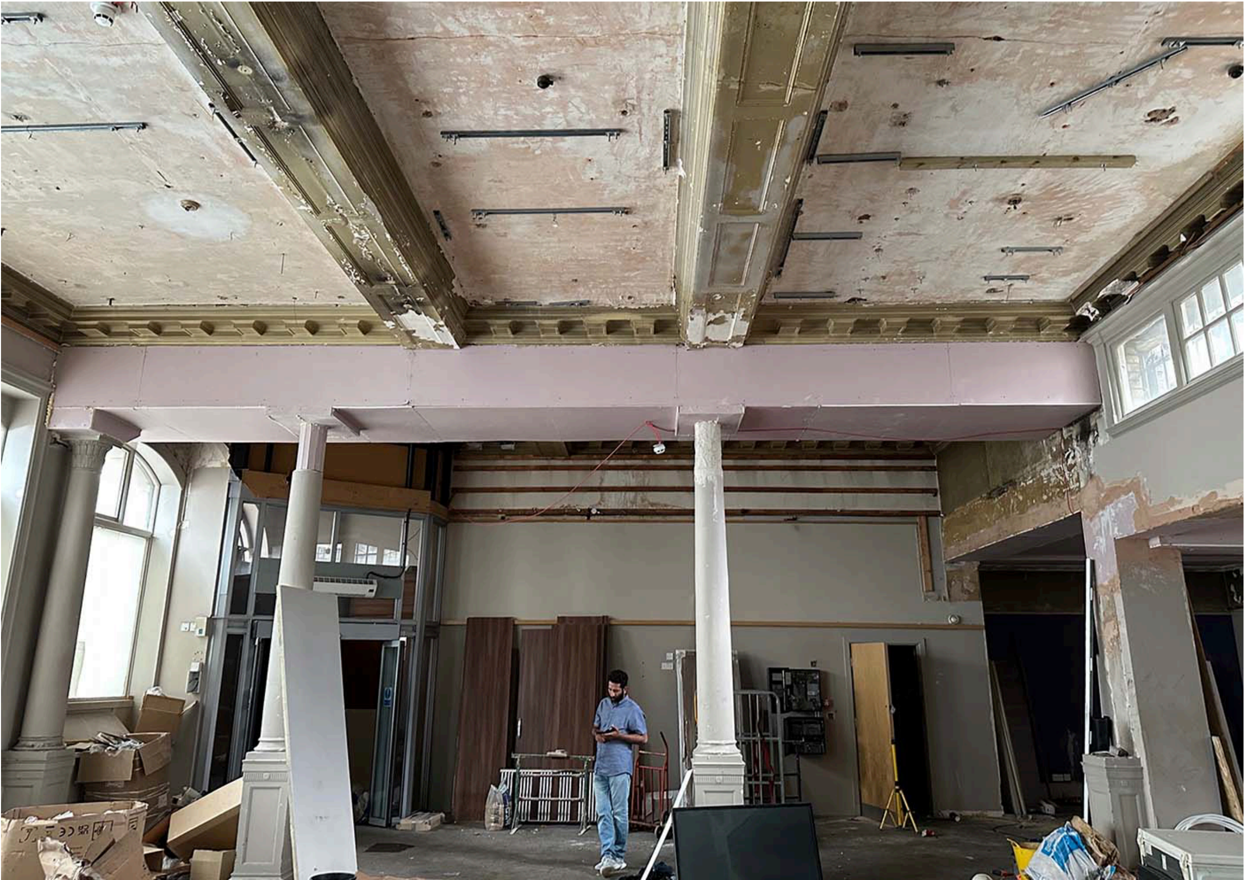
INTERNAL: VIEW NORTH
