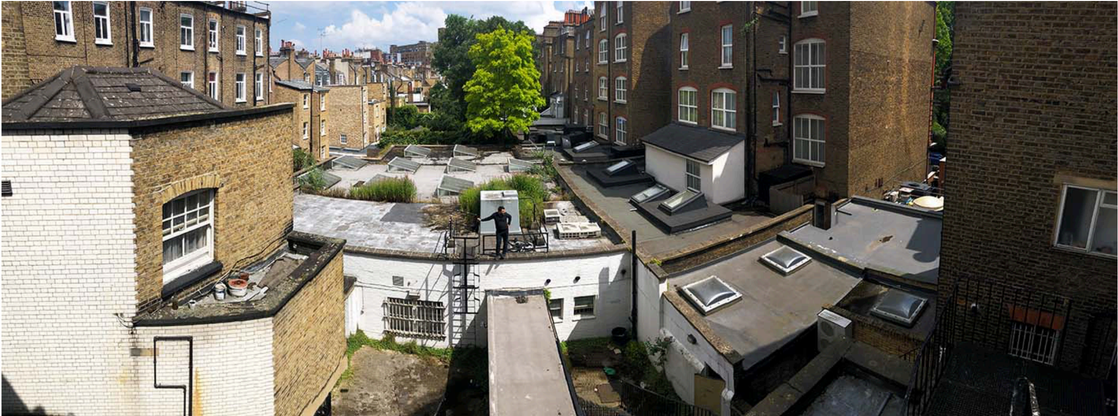
EXTERNAL REAR: LEVEL 2 VIEW EAST
